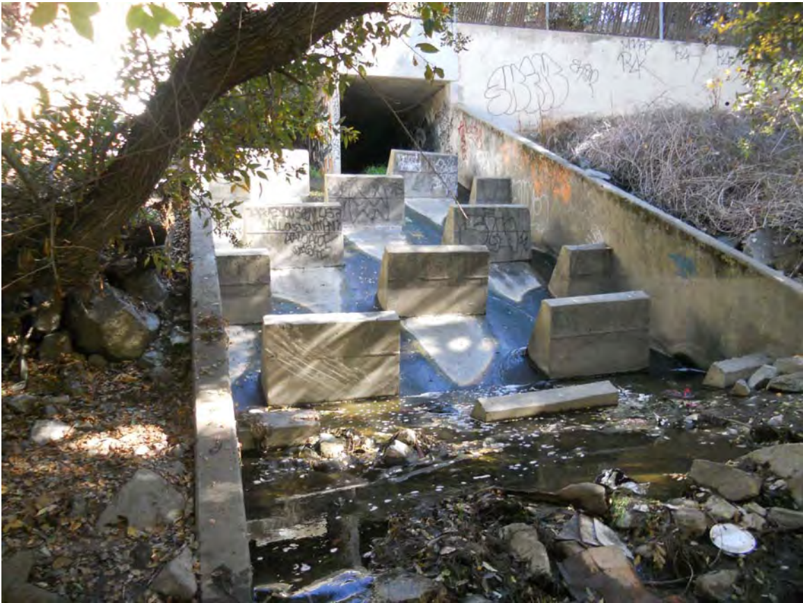
Barrier on water district property prevent steelhead trout from migrating to upper Silver Creek, trapping all steelhead trout within large homeless communities Depart. F&G warden Mark Imstall called numerous times 2002 to 2004. Photos DSCN1619 thru DSCN1624
